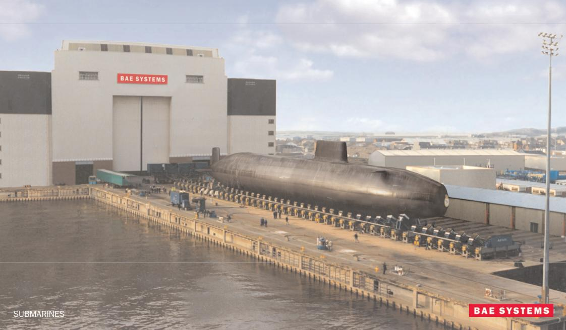
The Devonshire Dock Hall shipbuilding construction complex, with associated workshops and amenities, covers an area of 25 000m<sup>2</sup>. The height of the Hall at 51 metres was determined by the need for overhead cranes to clear the raised masts of nuclear submarines.
