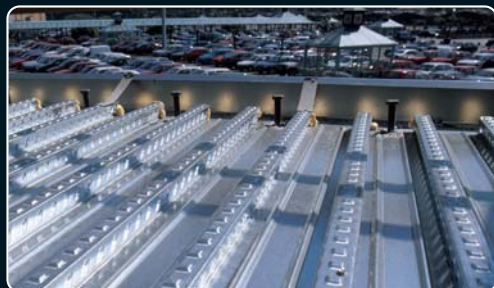
Multideck 50 profiled steel floordeck installation, Meadowhall Shopping Centre, Sheffield, UK
