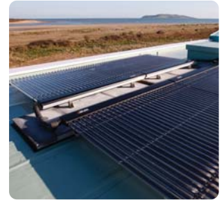
Thermomax DF100 collectors can be installed flat to suit any architectural requirements or building constraints
