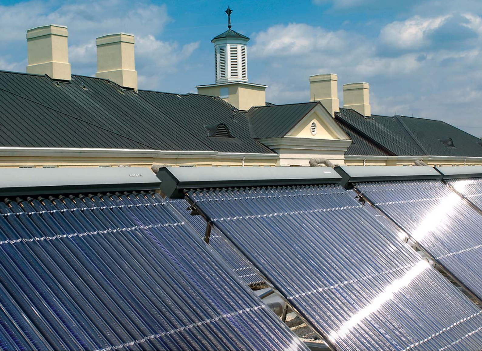
Thermomax advanced vacuum solar thermal system, University of South Carolina, USA
