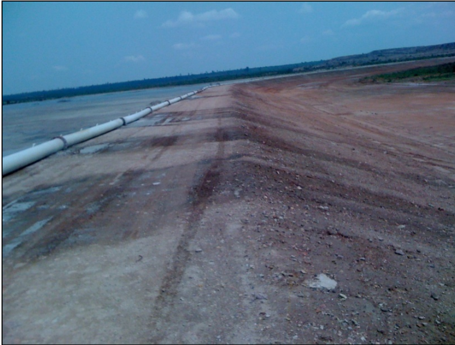
Figure 36: Western Flank of the KITD Starter Wall (looking south)
