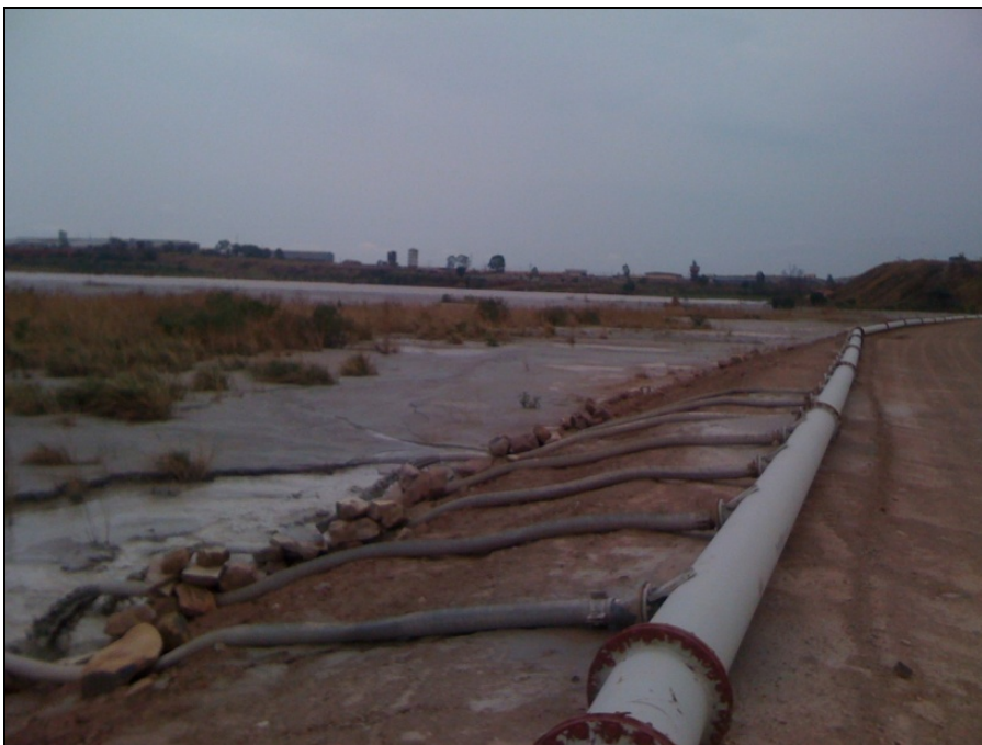
Figure 37: Spigot System Deposition on the eastern flank of the dam
