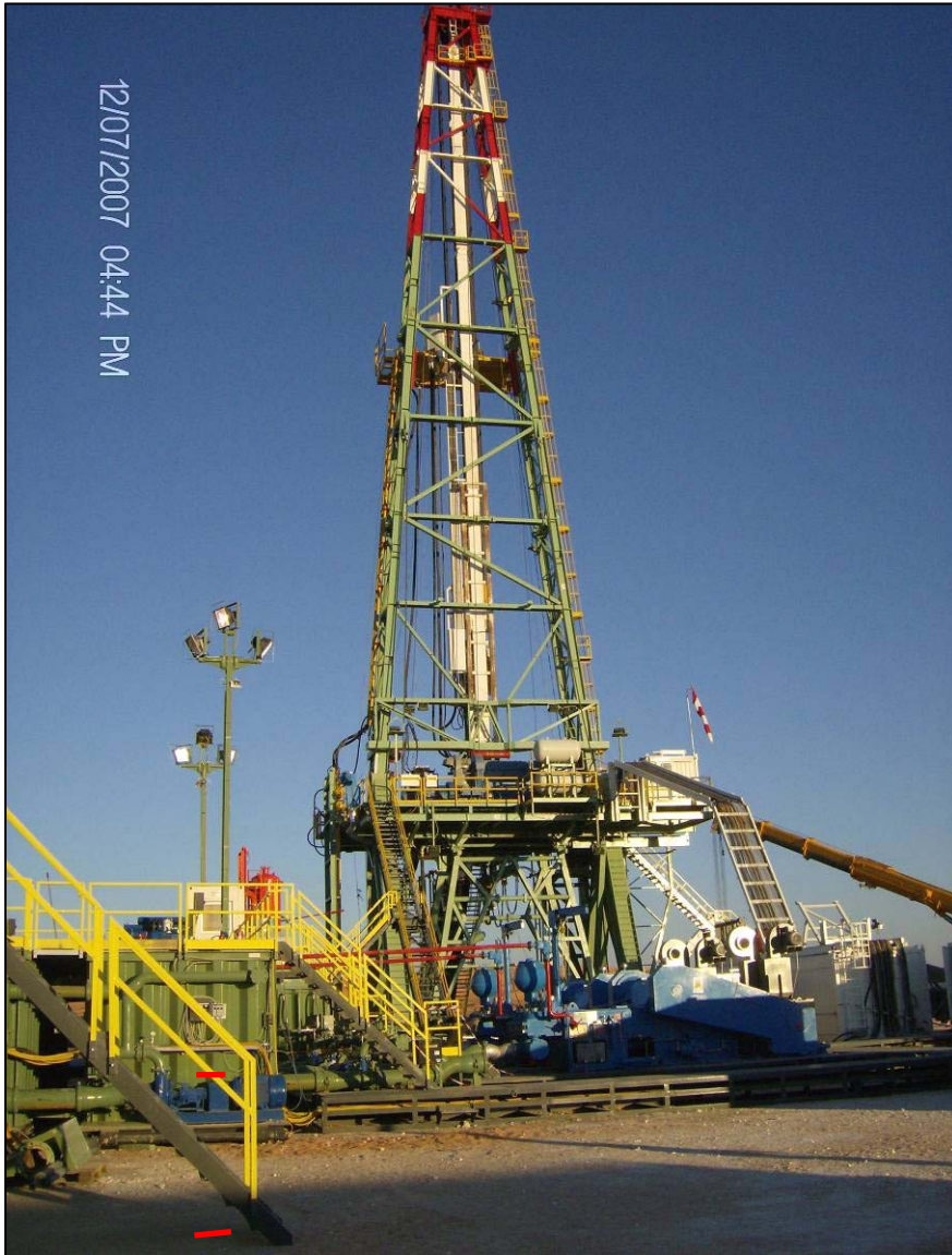
HBH-4 rig – photo courtesy of BG Group
