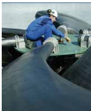
Howden Cooling Fan Howden SX-Series low-noise cooling fans are used in a wide range of cooling and ventilation systems that must meet strict environmental noise levels.
