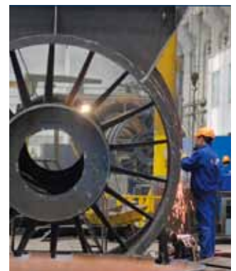
Fabrication of fan casing Flexible supply chains allow fabrication to be carried out in-house or at quality approved sub-contractors.
