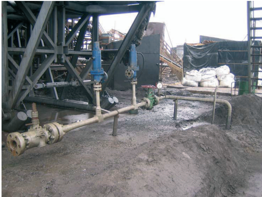
Flow line from Pirkovskoe-1 used for light oil production
