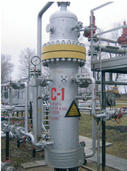
Close up of first stage separator C-1 in gas processing plant
