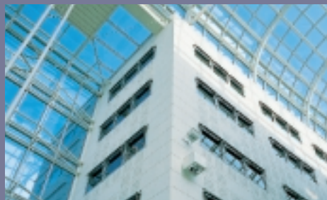
Acoustic internal wall linings
