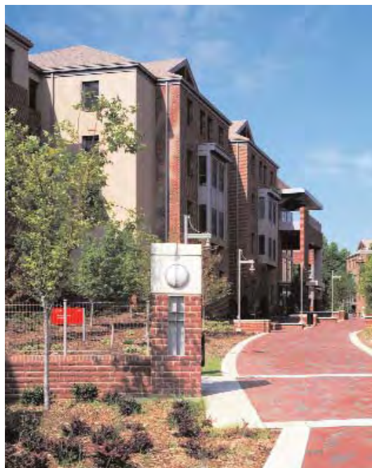
North Carolina State University, Wolf Village Complex in Raleigh, North Carolina
