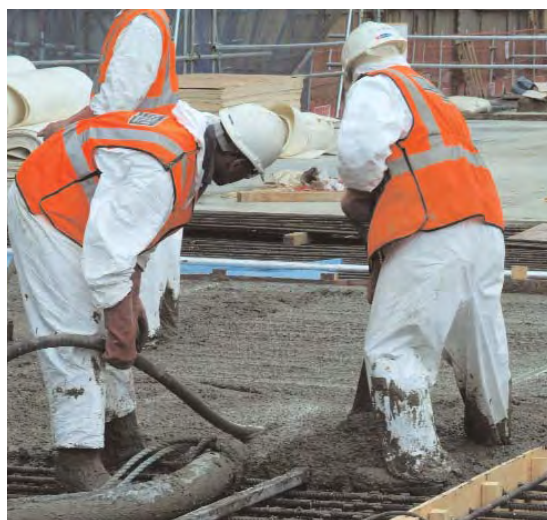
Schematic showing the full extent of the project. Below: laying concrete
