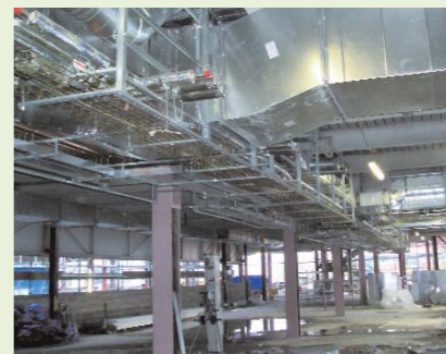
Addenbrooke's Hospital units in position
