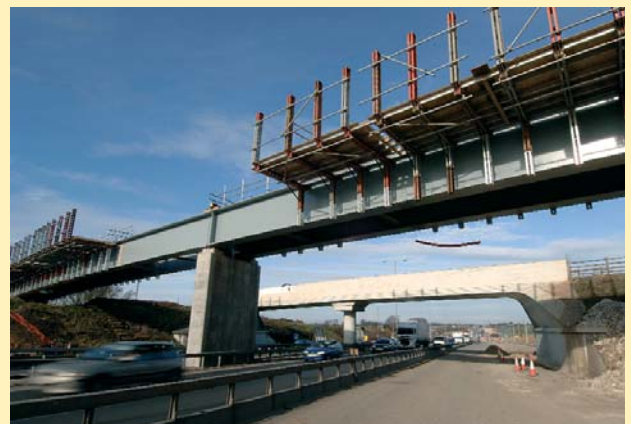
Future: the new bridge takes shape
