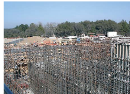
A forest of scaffolding surrounds the Roseville treatment plant project
