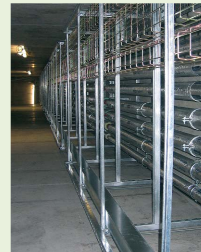
Pre-fabricated units ready for use
