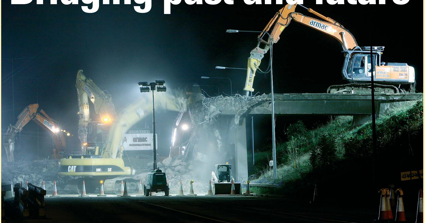
Past: The old bridge is demolished
