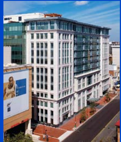
700 Sixth Street is a 12-storey office building in the Penn Quarter of downtown Washington DC. It was built by BBC's team in Washington, features over 300,000 square feet of office space, and achieved the prestigious designation of LEED Platinum.
