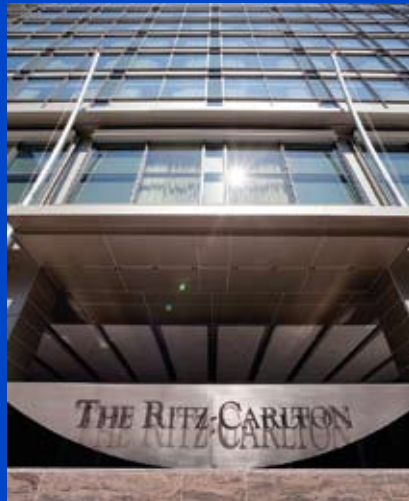
The Ritz-Carlton, Charlotte in North Carolina was completed by BBC and its team at RT Dooley in September 2009. The luxury hotel recently earned its official LEED Gold Certification, the first in the Ritz-Carlton chain to earn this level of green distinction.
