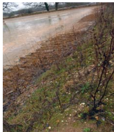
Willow mats are being used at Blashford quarry to drain silt ponds.
