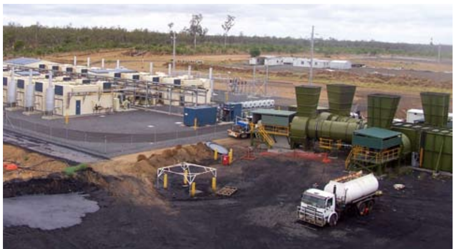
Anglo Coal Australia's Grasree underground mine, part of the German Creek mining complex, supplies coal seam methane to a 32 megawatt power plant owned and operated by Energy Developments Limited. Electricity generated by the power plant is sold into the Queensland grid
