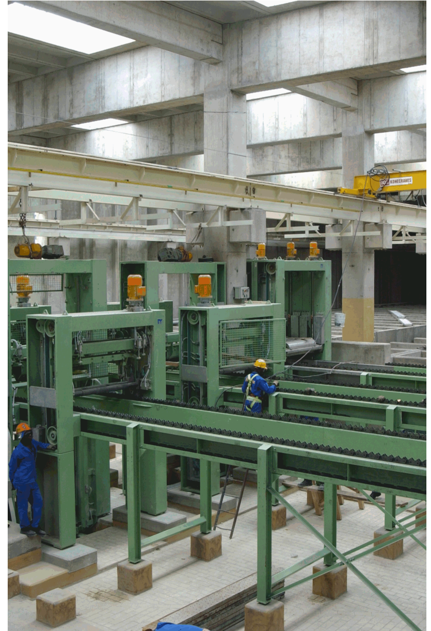
Construction of cellhouse
