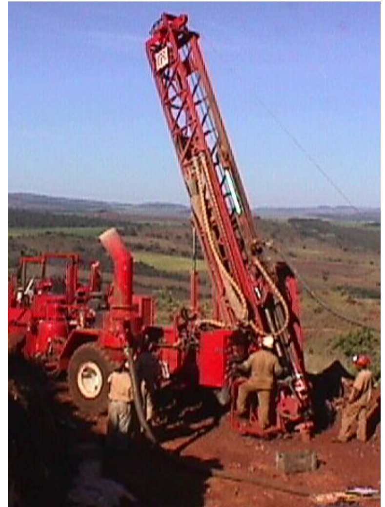
Drilling at Barro Alto
