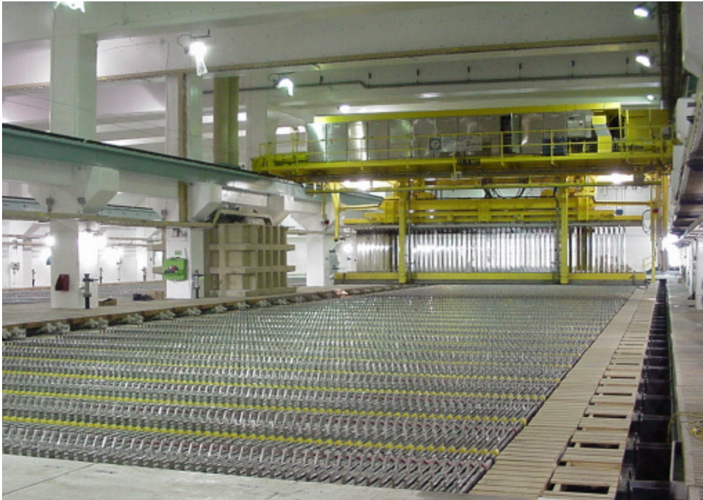
Inside the new cellhouse
