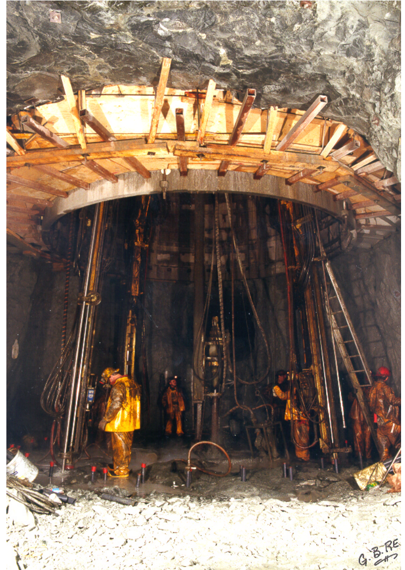
Shaft sinking at 777 mine
