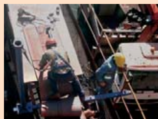
Left: A foreman and two operators at Sishen, who investigated the risk to personnel repairing conveyor belts, have developed an overhead hook-up system which can be attached to any conveyor structure.
