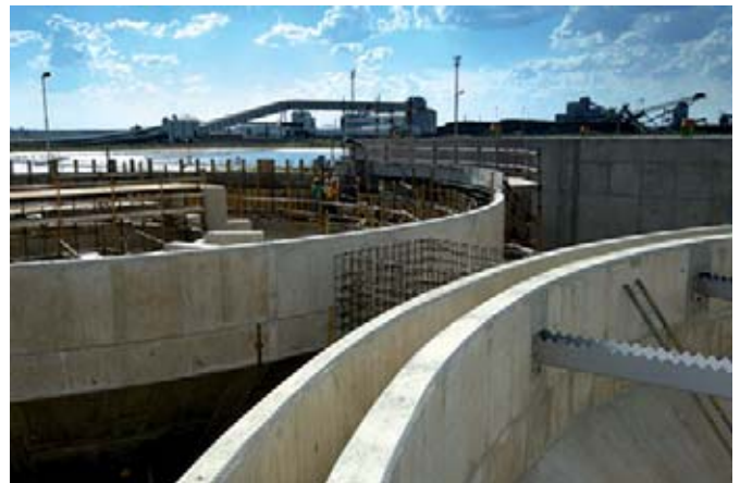
Above: Construction of the Emalahleni water treatment plant nearing completion.
