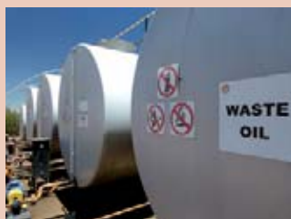
Left: All used and spilled oil is collected into these containers before being sent away for recycling.
