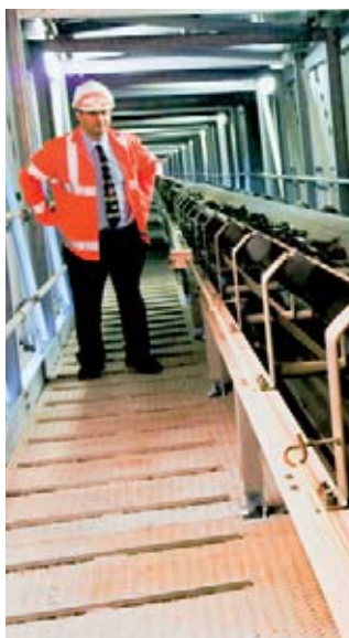
Left: Hasan Bobat, fuels development engineer at Tunstead, standing next to the conveyor belt.
