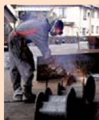
Left: Welding fume exposure is a common industry hazard.
