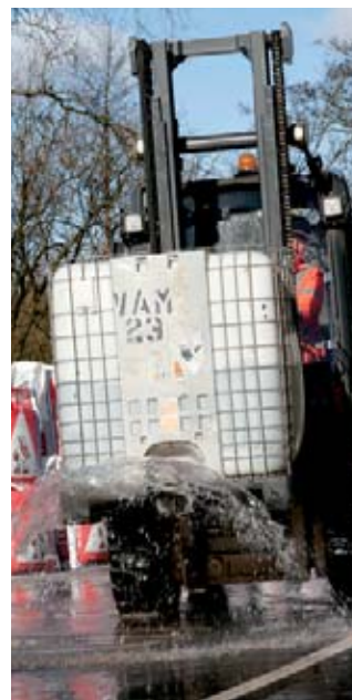
Above: A forklift is used to distribute rainwater collected off the buildings at Tarmac's Chatburn, UK, site with a saving in water and costs.
