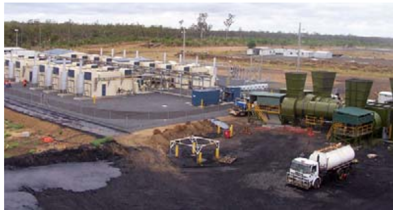
Above: Anglo Coal Australia's Capcoal power plant at German Creek mine, is one of Queensland's first electricity generators to be fuelled by coal seam methane.
